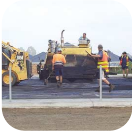
The court under construction at South Colac
