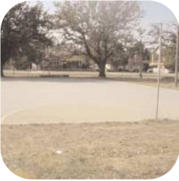
Before: the substandard surface
