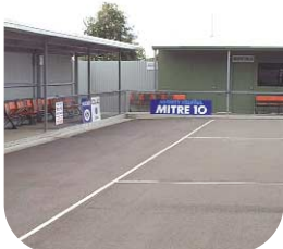
The new facilities at South Colac
